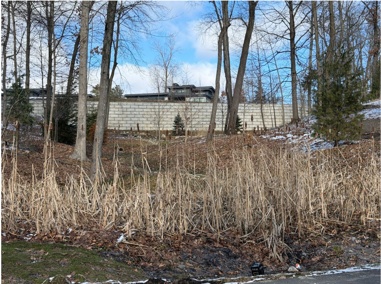
2026 Retaining Wall view from Thornapple River Drive
