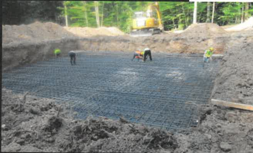
Pic Above: New Tower Foundation
