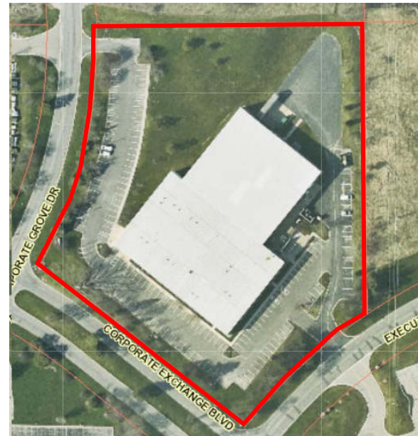
Above: current site conditions
