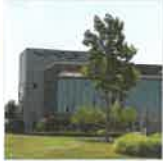
Auburn Hills Facility Sales HQ Auburn Hills, MI
