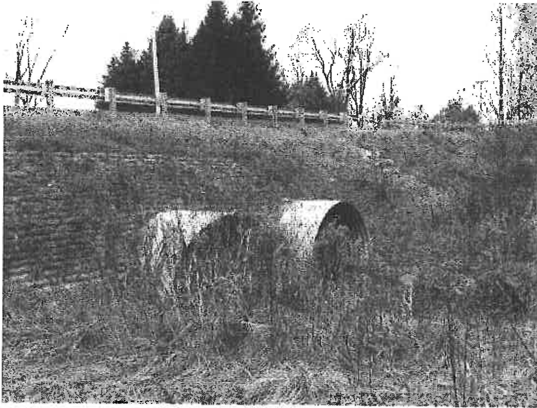
Downstream side of crossing. Photo from November 2009 Inspection Archive.
