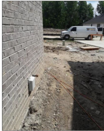
Clear pathway from meter location to street.
