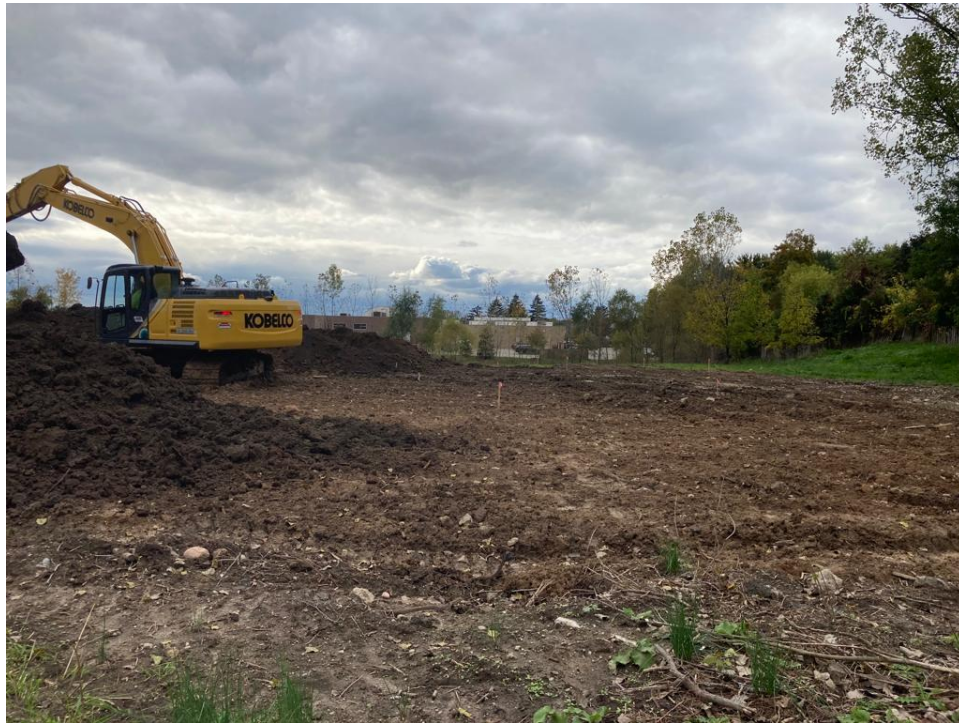
10/22/21 – West side of the former stockpile, stockpile removed (facing west)
