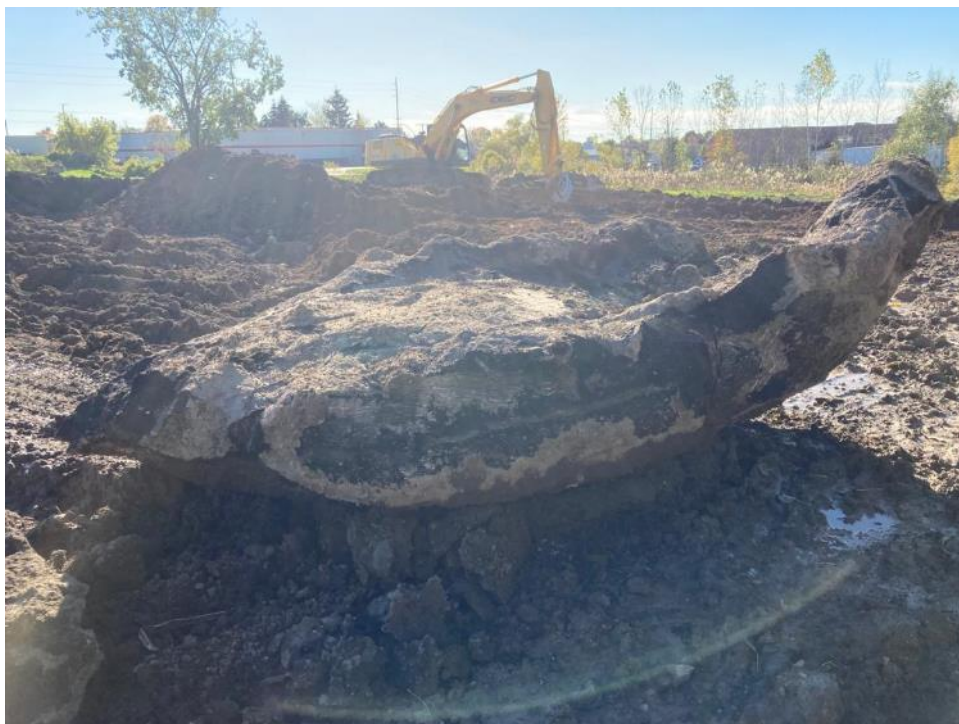
10/26/21- Concrete chunk discovered through northern side excavation (facing southwest)
