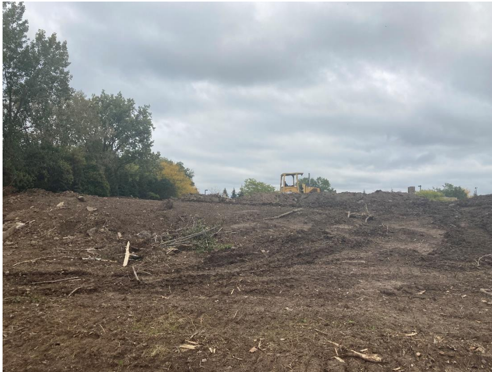
10/5/21 – West side of the former stockpile, removal in-progress (facing east)
