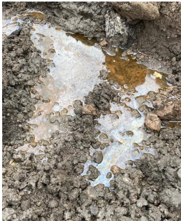
11/4/21 – Sheen observed near east wall of the basement excavation. Soil and groundwater sampled under Grant Assessment Task.
