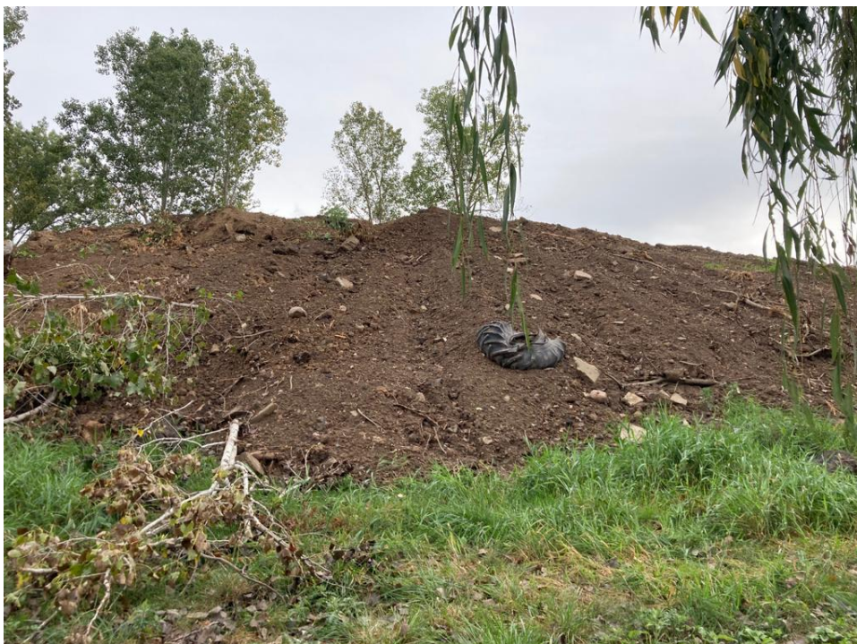
9/22/21 – West side of the former stockpile, removal in-progress (facing east)
