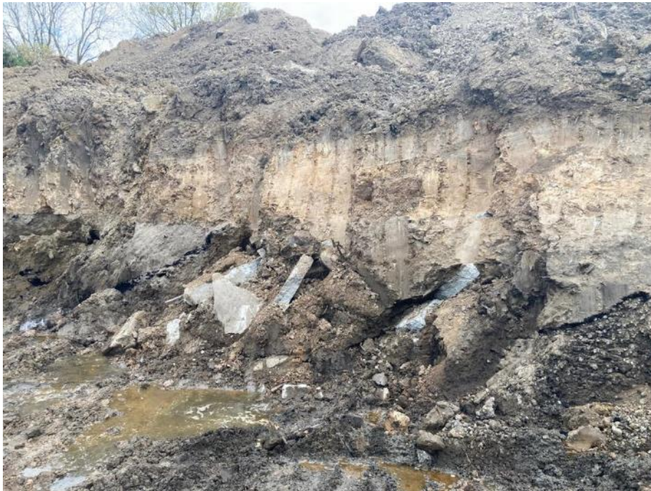
11/4/21 – East wall of the basement excavation (facing east)
