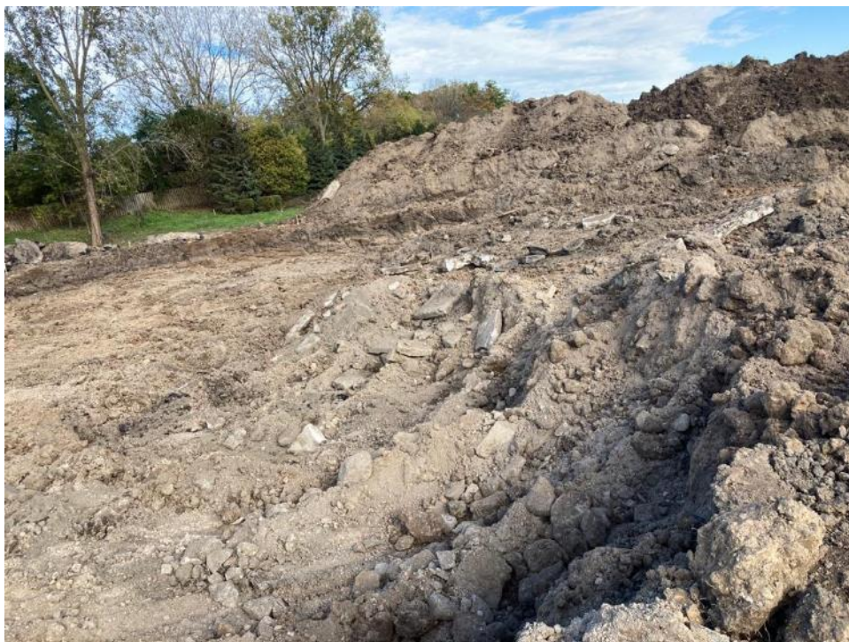
10/28/21- Fill material encountered to the depth of 6 feet (facing northeast)
