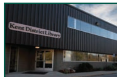
KDL SERVICE AND MEETING CENTER 814 West River Center Dr. NE Comstock Park, MI 49321
