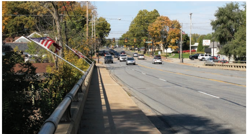
Cascade Road bridge over the Thornapple River, looking northwest. Enhancements will include a physical barrier to separate the pedestrian lane from traffic, a higher outer railing, and year-round lighting.
