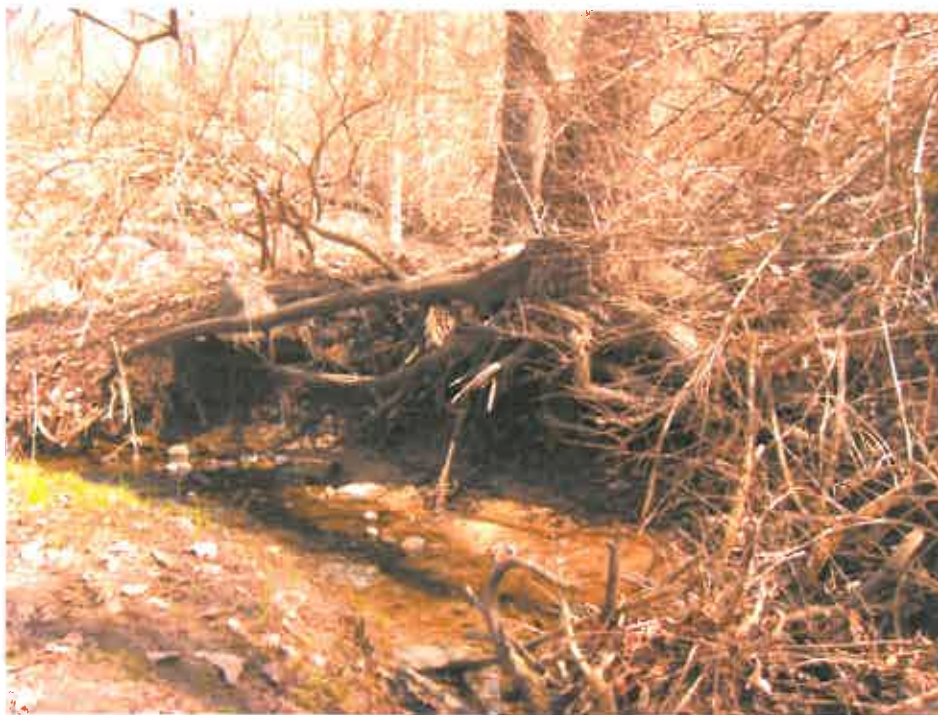
Bank erosion and undercutting of trees (channel to be relocated/stabilized)
