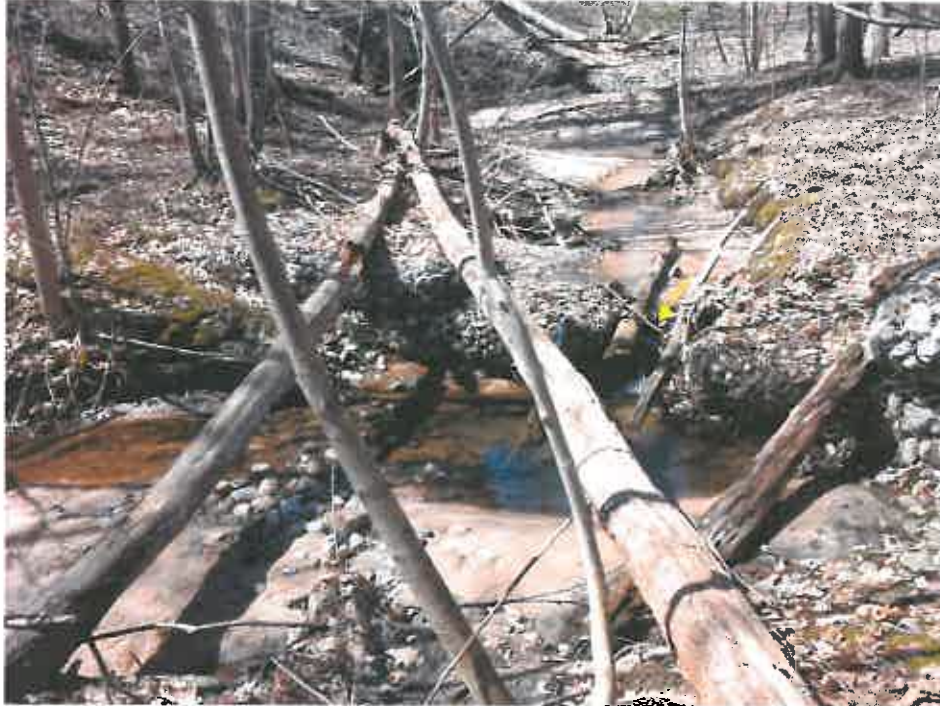
Typical unstable grade; sediment in Drain (install grade control structure)
