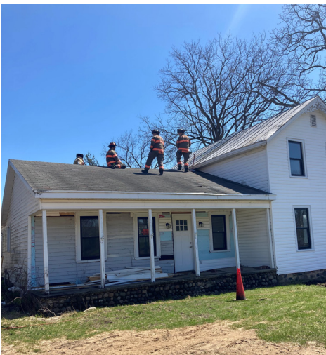
TRAINING AT FF. LANCE KORHORN'S HOME BEING DEMOLISHED
