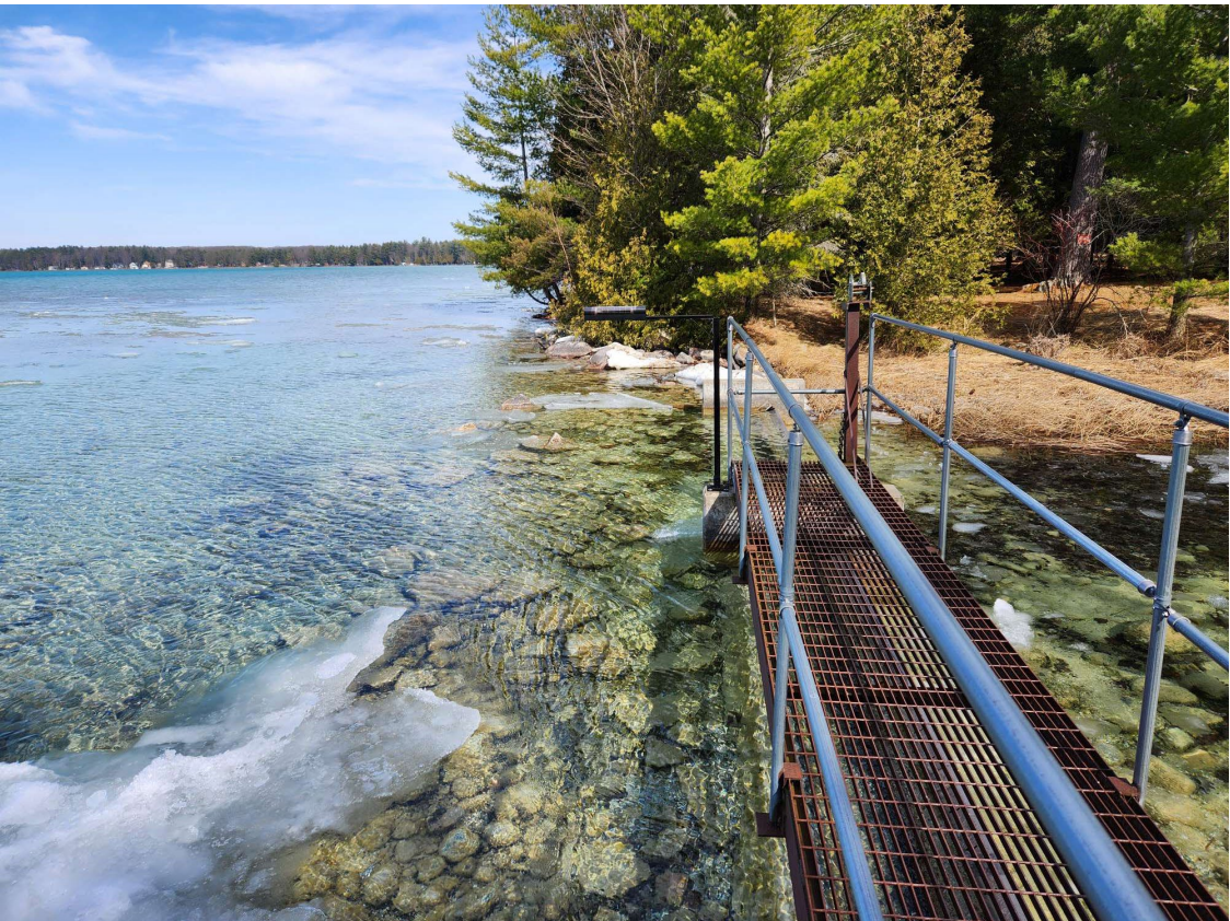
Monitor elevated above the high water line:
