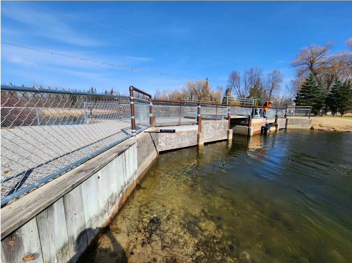
Monitor flush with wing wall:
