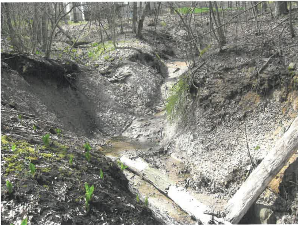
Ravine erosion downstream of storm outfall—Tammarron District
