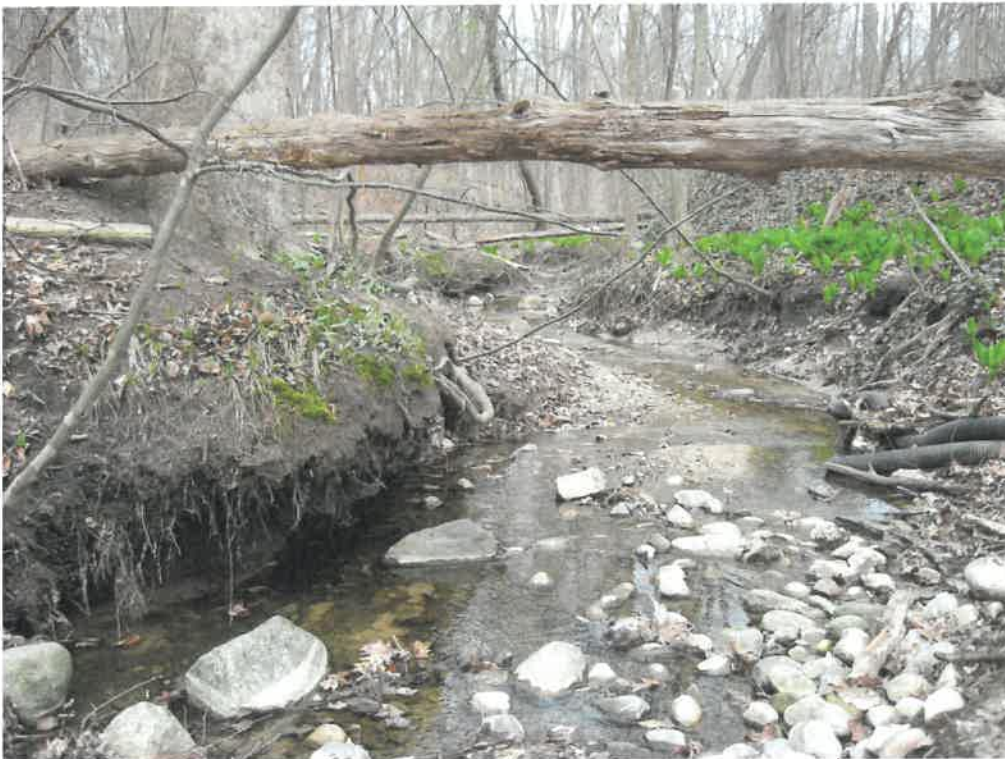
Unstable pattern; downcutting; poor floodplain connectivity; Burger 1 District
