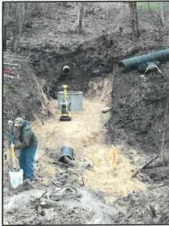
New catch basin installation - Thornapple Hills Drain (Sentinel drainage district) February 2017
