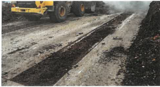
The 100 foot by 200 foot, 2 zone composting pool has pipes in the trenches of the aeration zones (above). The system runs in both positive and negative aeration modes.
