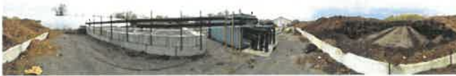
Panoramic view of Country Oaks Landscape Supply, showing, from left to right, the end of the composting pad, new greenhouse, biofilter, CAHR unit, the shop and sales building, and back to the composting pad and recessed channels. Photo by Jason McCune-Sanders, Agrilab Technologies Inc
