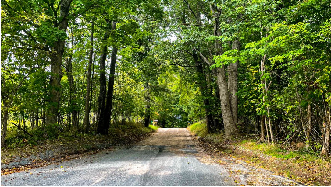
Looking north on Alaska Avenue at the point where the paved street becomes gravel. The gravel cross-section is about 20' wide.
