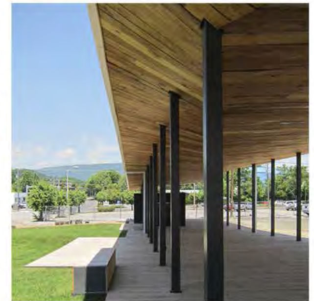
OPEN AIR PAVILION
