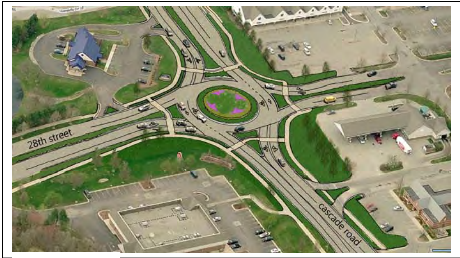
Courtesy of Progressive AE
