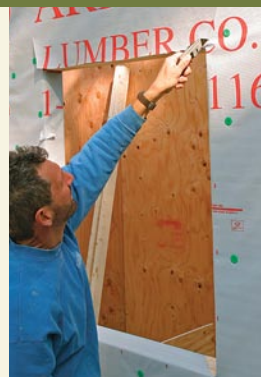
Staple the tabs down, then cut the top tab.
