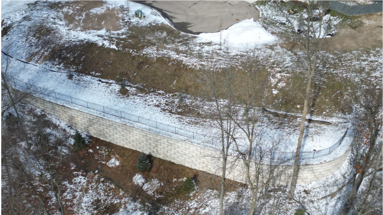
2026 Aerial of Existing Retaining Wall
