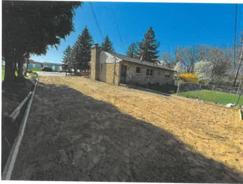
Figure 3 Driveway from Garage to House
