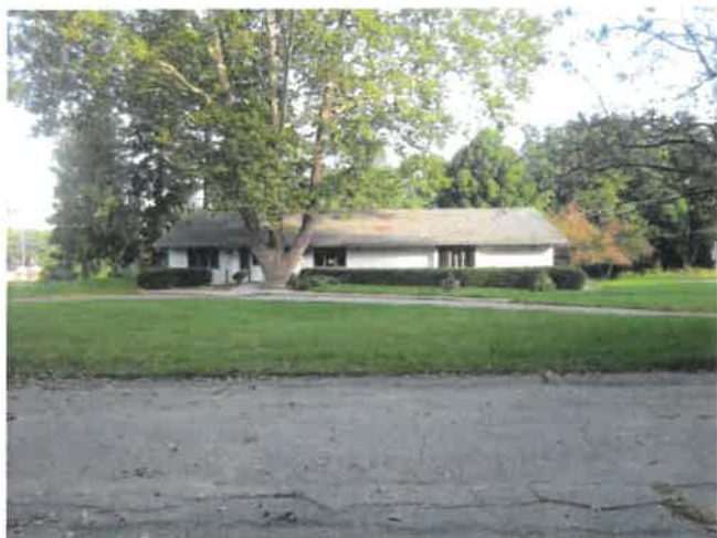
The church building facing northerly
