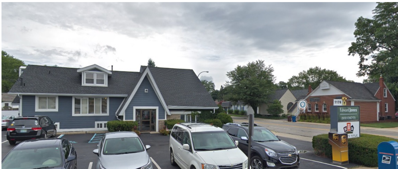
South Main Street in the City of Plymouth, MI is an example of horizontal mixed-use development. Note the sidewalks, streetlamps, buried utilities, minimal signage, street trees, reduced building setbacks, and other similar placemaking features.
